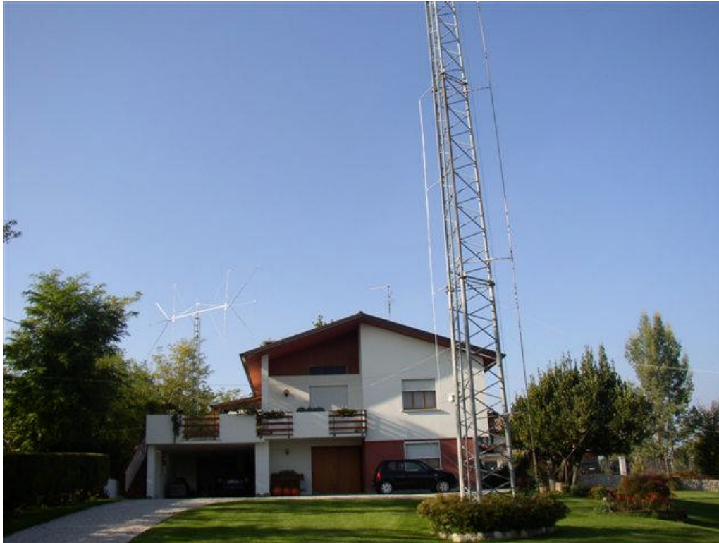
The last picture of the Waller Flag .....before dismantling, after one month tests. The left rod on the TX tower forms the detuning section. On the right the gamma rod.
