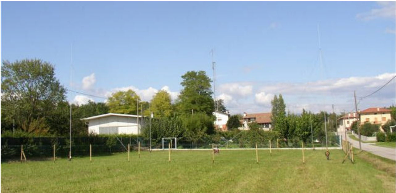
Complete view of the 4 square Rx array installed on the fenced 26 x 29 meters lot.
