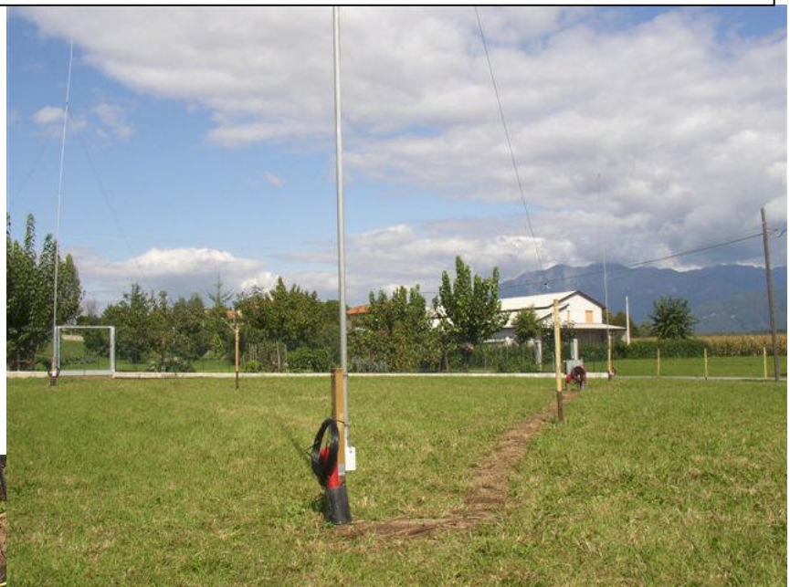
Complete view of the 4 square Rx array installed on the fenced 26 x 29 meters lot.
