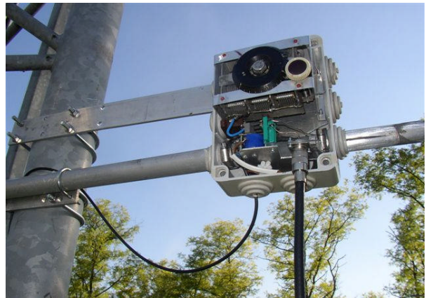
Fig.6: the detuning capacitor box
