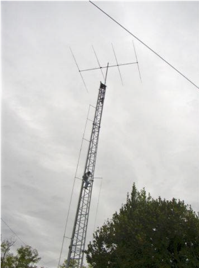
Fig.5: IV3PRK installing the detuning loop
