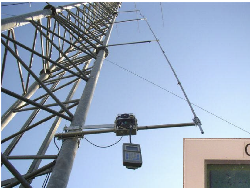
Fig.7: The full tower detuning loop
