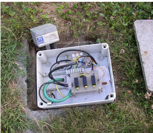
The Pennants central box ready to be buried with a K9AY preamplifier
