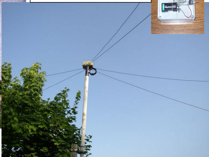
The Pennants switching box of the southern group with the added common mode choke.
